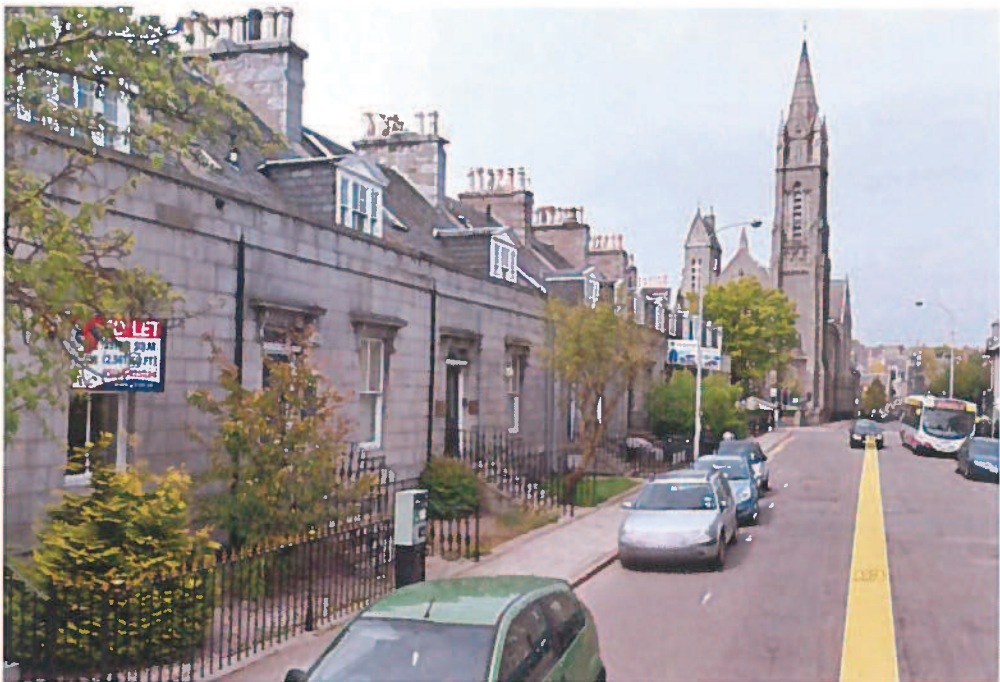
Figure 2: Photograph of Terrace along Albert Street
